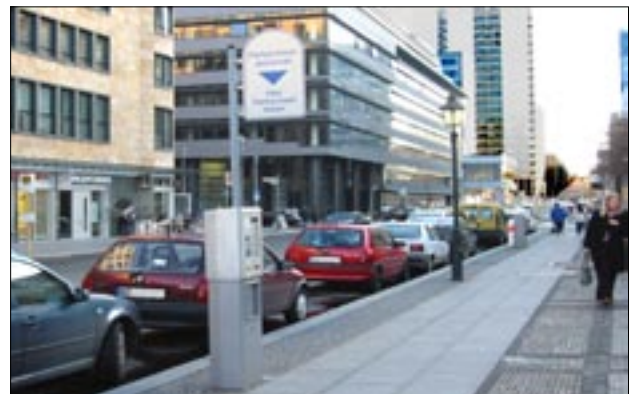
Installation in Berlin.
